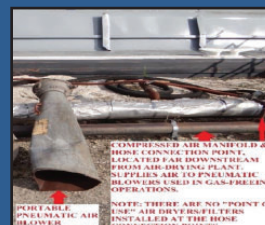
Not installing "point of use" air dryers at hose connection points for pneumatic air blowers (left photo) and attaching air blower bonding clamps to painted surfaces instead of bare metal (right photo) can lead to dangerous static build up
